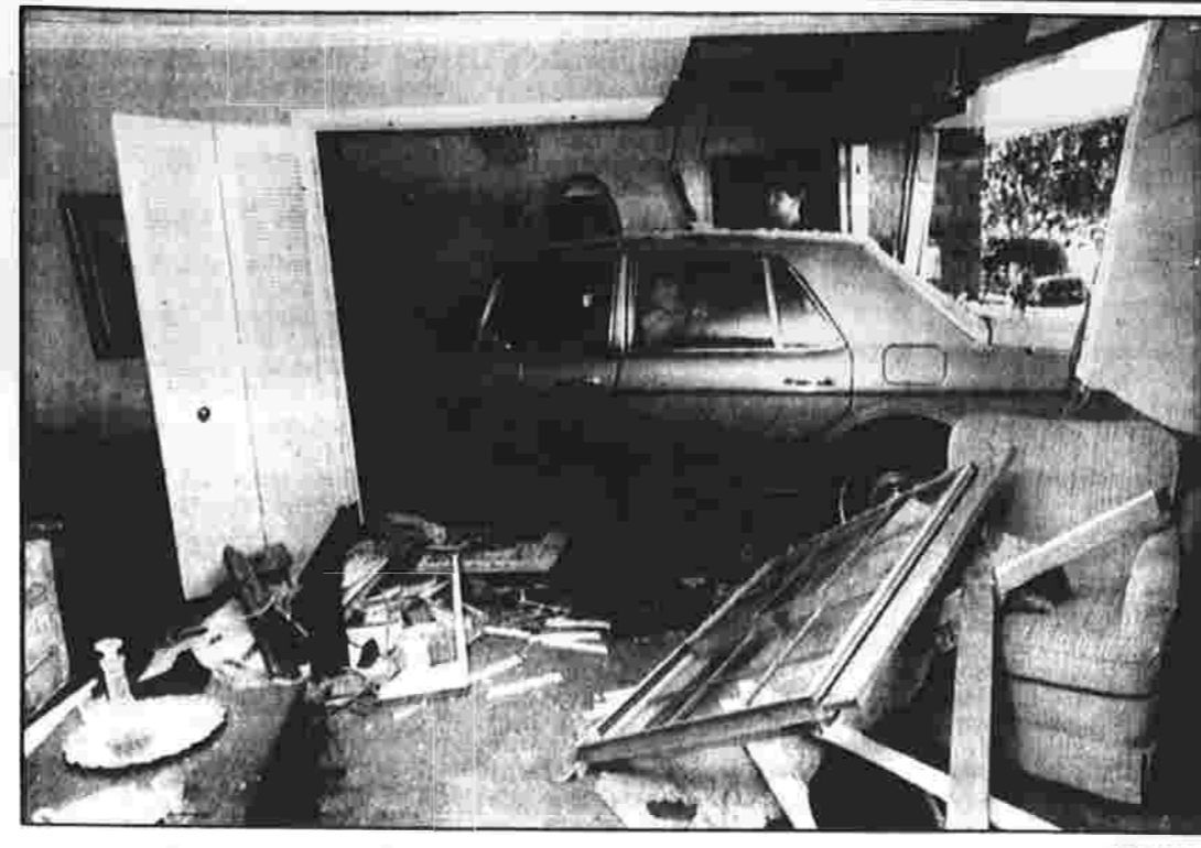
UNWANTED COMPANY — A 1988 Rolls Royce sits in a New Orleans house after crashing through the wall Tuesday. Police said the driver, Jeanette Maranto, 83, told them the steering wheel locked,
